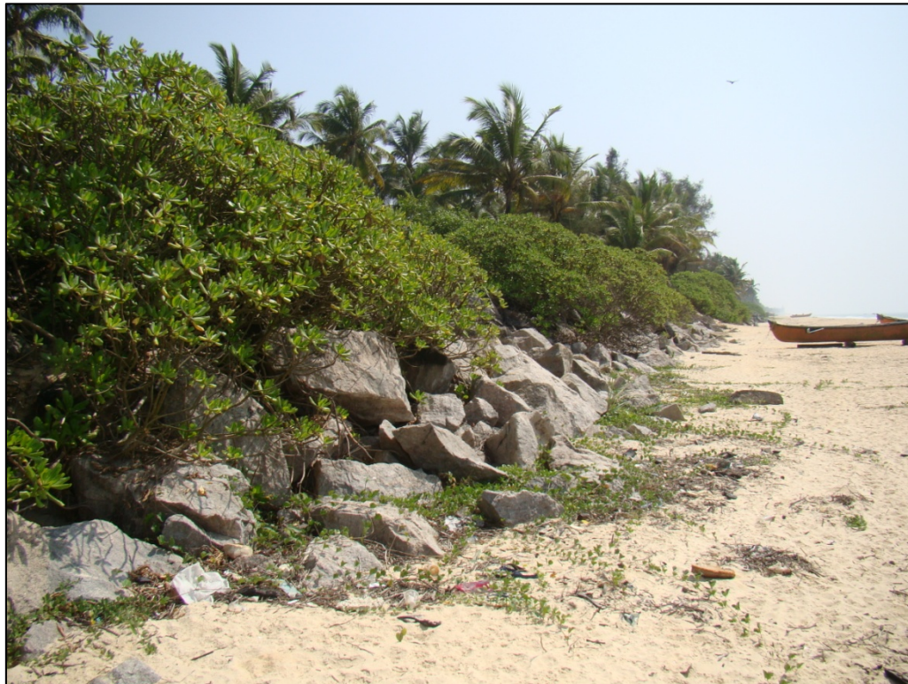
Plate 32: Sea wall covered with vegetation indicating a stable shoreline north of Mukka (48K16SW) along Southern Karnataka coast
