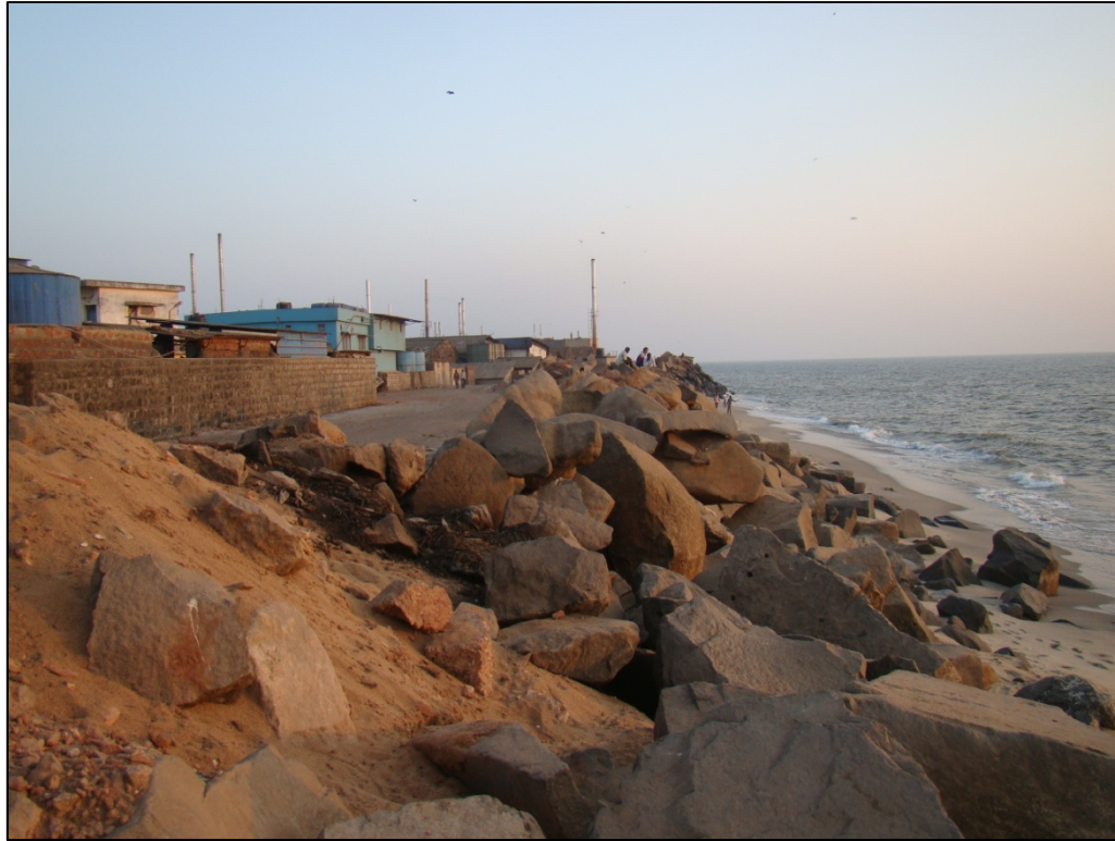
Plate 37: Sea wall to check coastal erosion at the southern bank of Netravati river (48L13SW) along Southern Karnataka coast
