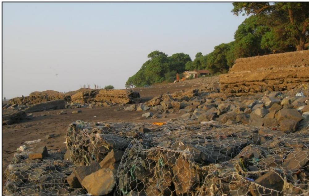
Plate No. 48: Collapse of Sea wall near Umarsadi, south Gujarat (Map Sheet no. 46D14SE)
