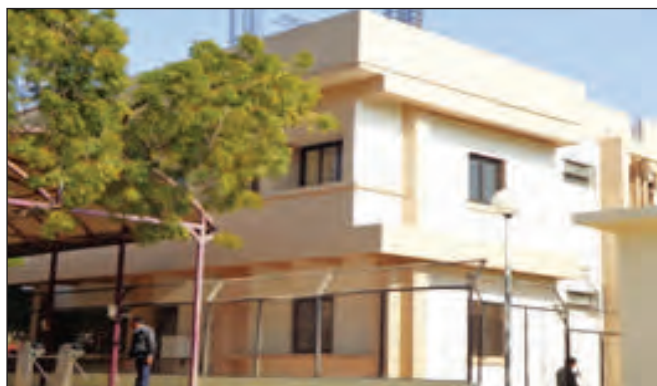
Horizontal extension of building No.30
