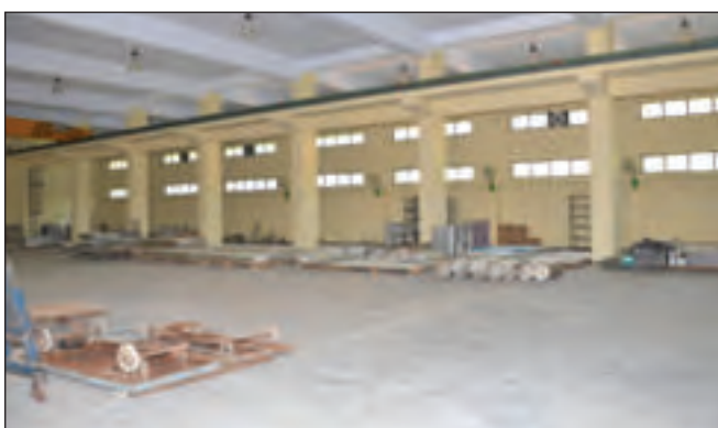
Interior view of high bay area of MMFS
